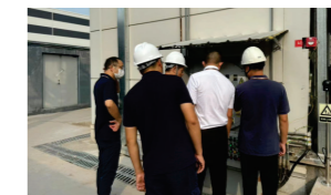
Management-led Safety Inspection
