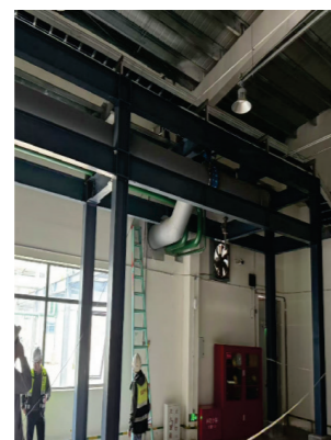
Technical Renovation of Air Separation Station 1
